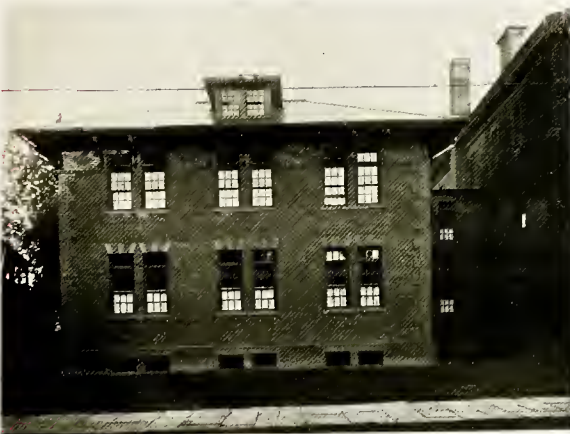
Addition to Home for Friendless Children South Franklin Street
